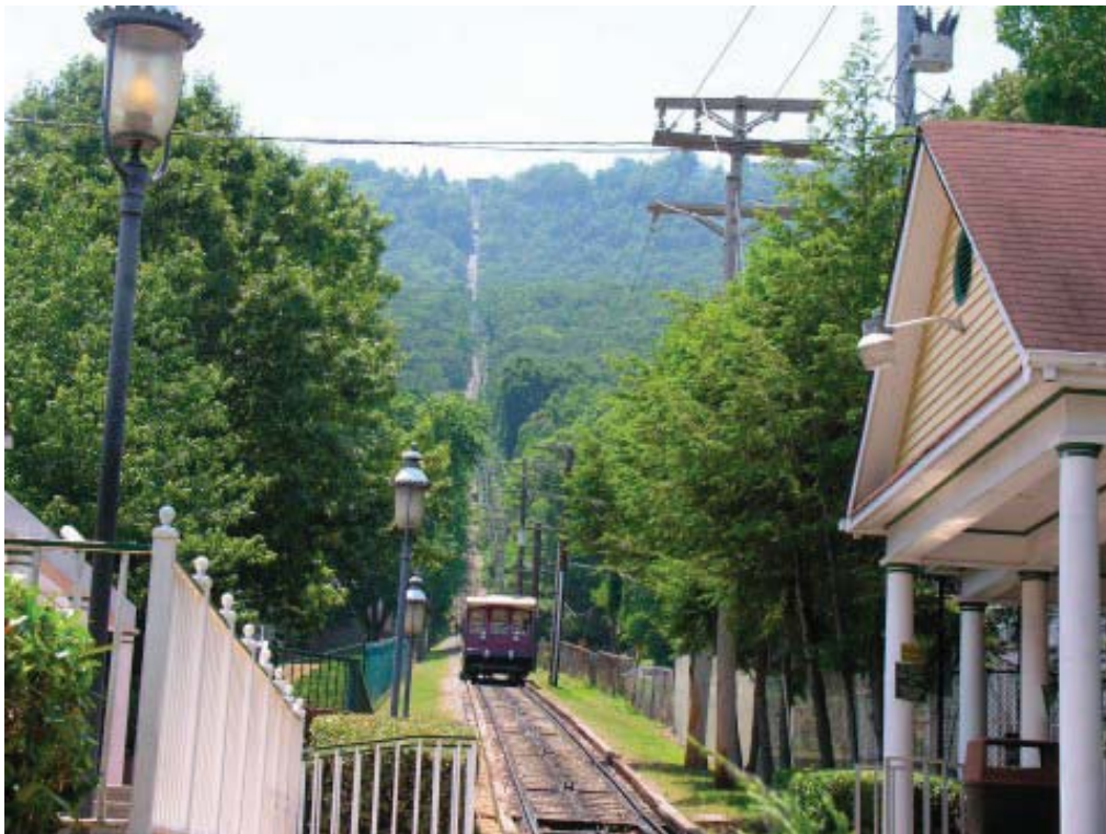
Incline RR Car Unloading Point
